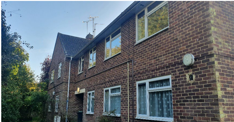
North east elevation of the building, windows facing the eastern boundary of the site.
