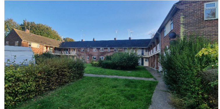
North/ front elevation of the existing building and front garden area.
