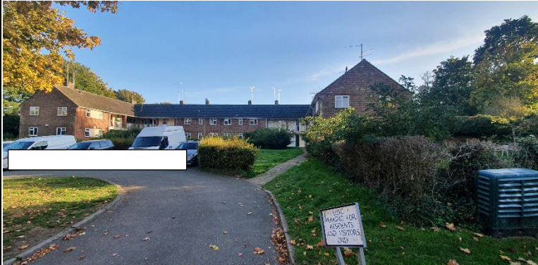
North/ front elevation of the existing building and parking area.
