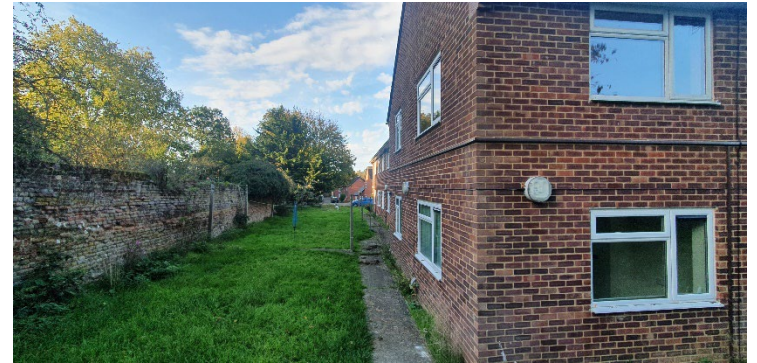
West elevation of the building, wall boundary of the park.
